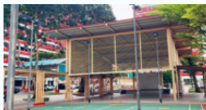
14 Improvement of shade through installation of louvers at hardcourt opposite Block 9 Toh Yi Drive
