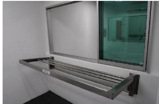
The retractable clothes drying rack with poles extended within the frame to dry laundry (left) and with poles retracted when hanging or retrieving laundry (right)
