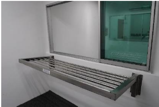
The retractable clothes drying rack with poles extended within the frame to dry laundry (left) and with poles retracted when hanging or retrieving laundry (right)
