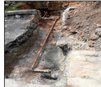
Stage 2: Transferring connection to the houses
