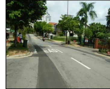
Stage 1 : Laying new pipes and temporary reinstatement of the trenches at the end of the day
