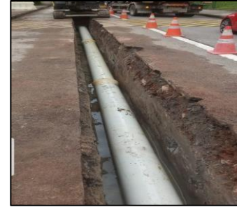
Stage 1 : Laying new pipes and temporary reinstatement of the trenches at the end of the day
