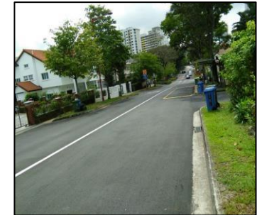
Stage 3: Full reinstatement of the road lane
